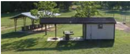
This picture depicts the old shooting shack in the foreground and the newly built benchrest line in the background.
